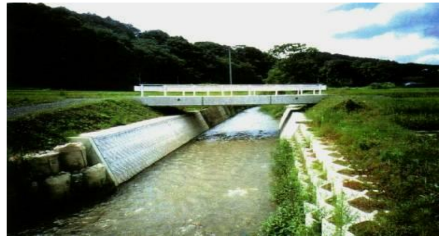
PC単純床版橋で復旧
