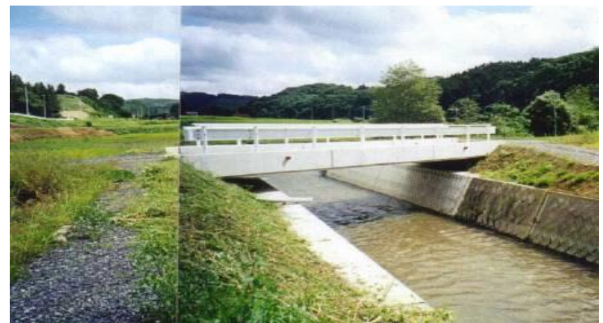
PC単純床版橋で復旧
