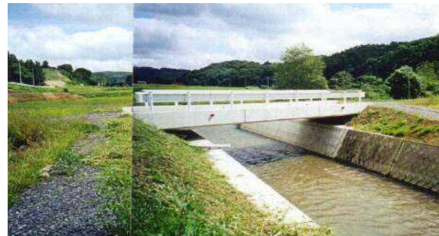
PC単純床版橋で復旧
